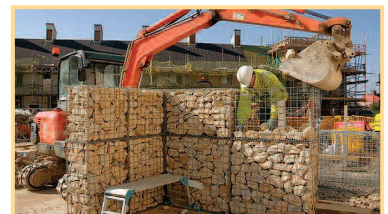
Single cage gabion wall with landscaped backdrop
